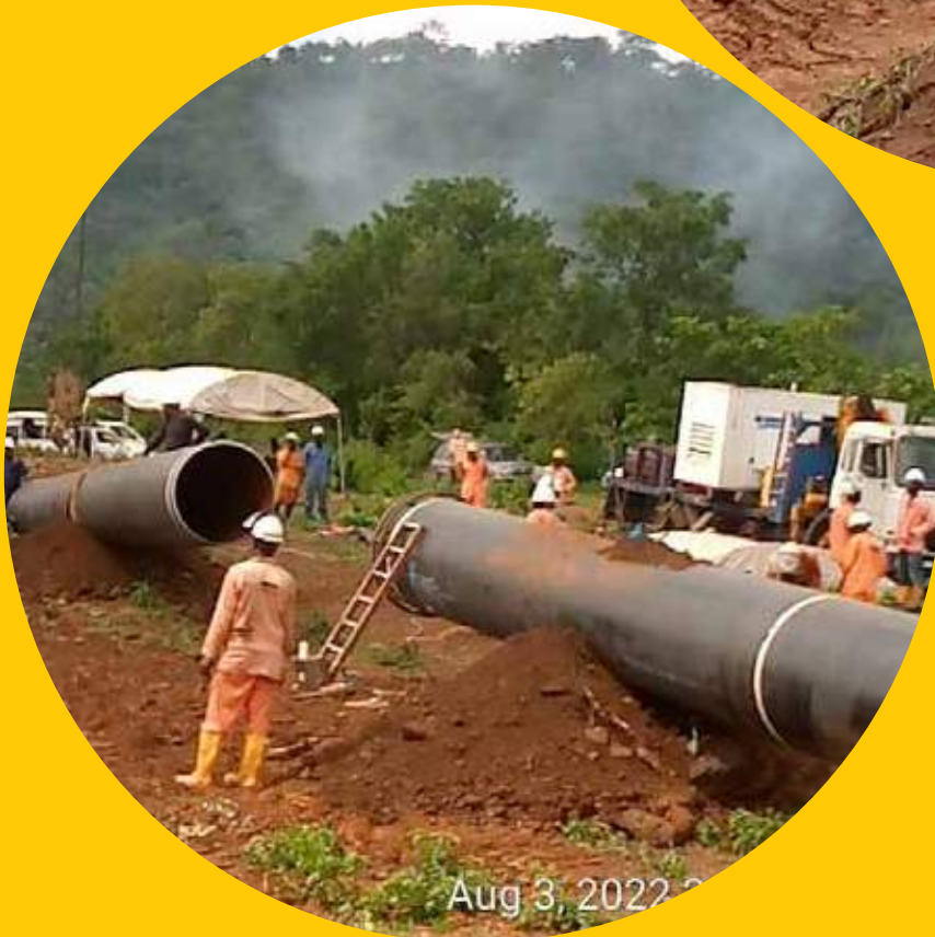
Fit up of 40 Inches AKK Pipeline project
